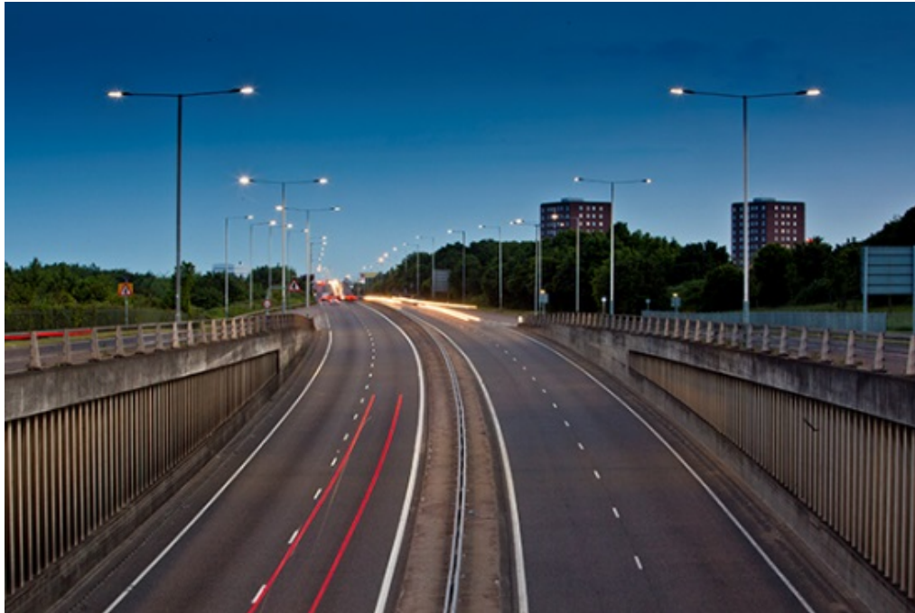
Figure 1 Example of lighting: a road and underpass
